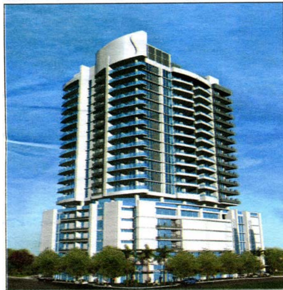
Strada 315 comprises ground-floor commercial space, plus five floors of parking and 13 floors of lofts.
